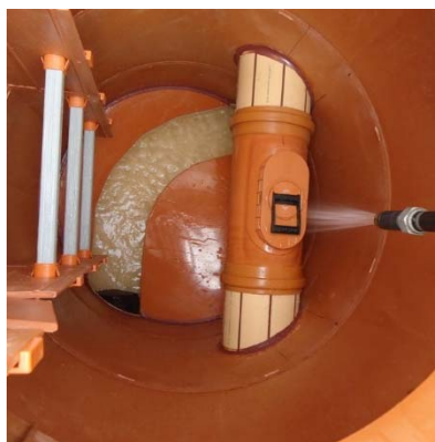
Figure 4 : Chamber watertightness control
