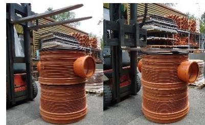
Insertion of the extension (point 5)
