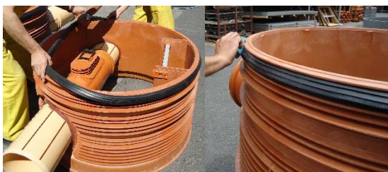
Insertion of the sealing joint (point 4)
