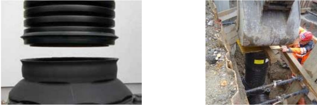
Figure 2: Installation of the extensions
