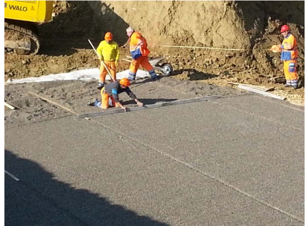
Figure 2 : Laying modules on the geomembrane and geotextile
