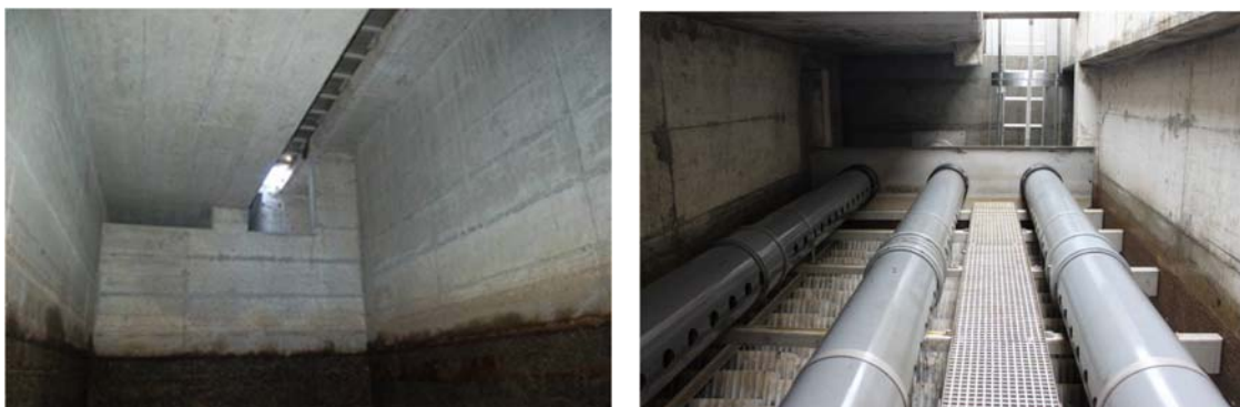
Figure 1 : Before and after the installation of basins with lamellar settling systems
