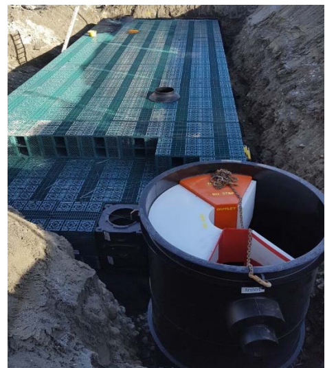
Figure 2 : First Defense® upstream of a Rigofill® system
