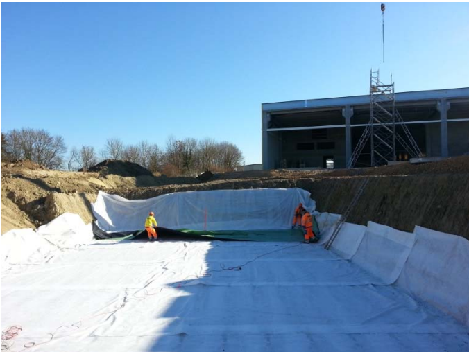
Figure 3 : Realisation of basin inlets/outlets
