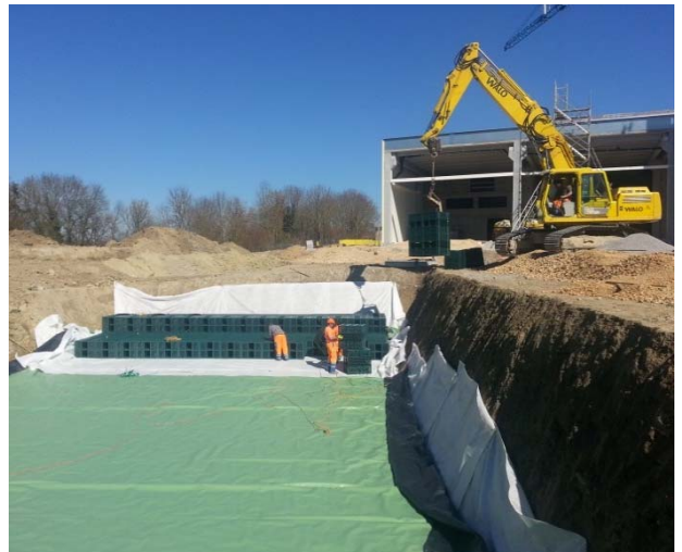
Figure 4 : Backfilling of the retention basin
