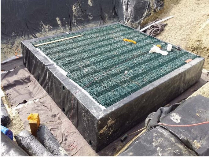
Figure 9 : First welding step to ensure total watertightness
