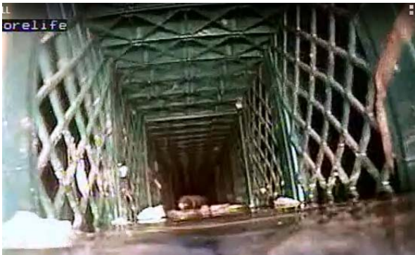
Figure 1 : Inspection before cleaning Rigofill® Modules containing large amount of macro-waste (dirty basin)
