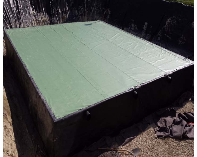
Figure 10 : Totally watertight basin
