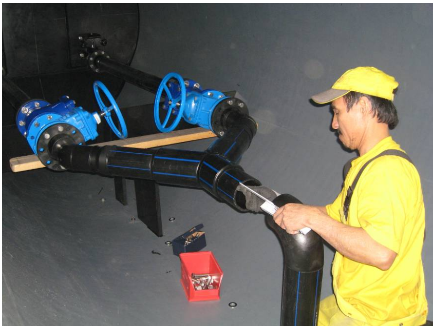
Mounting the discharge outlet in PE pressure
