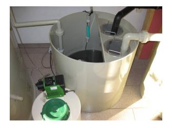
**In-line treatment** (Coagulation / pH neutralisation / Flocculation)
