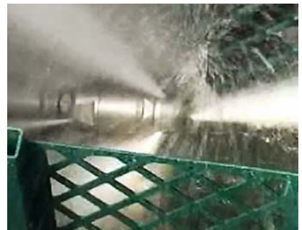
Figure 4 : Hydrocleaning inside inspection tunnels
