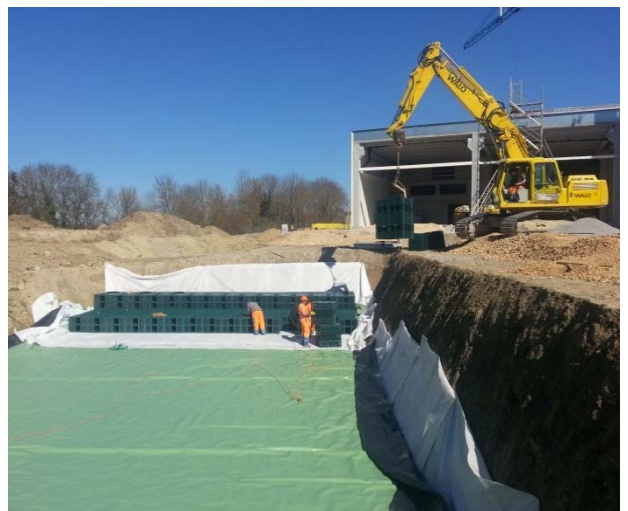
Figure 4 : Backfilling of the retention basin
