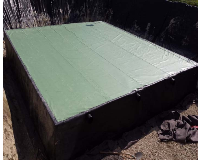
Figure 10 : Totally watertight basin
