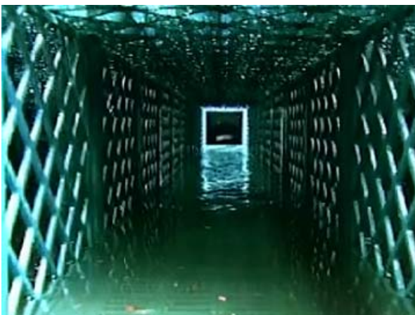
Figure 3 : Inspection of a Rigofill® basin after hydrocleaning via the cleaning passage
