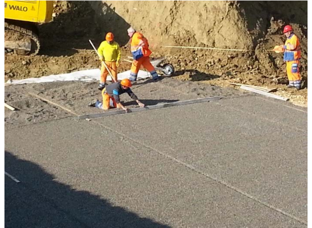
Figure 2 : Laying modules on the geomembrane and geotextile
