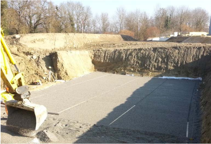
Figure 1 : Levelling of the excavation bed
