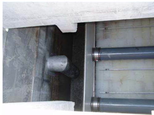
Figure 8 : Settled water channel
