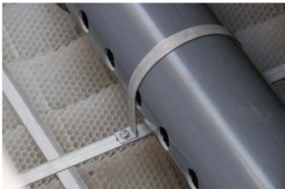
Figure 7 : View of the lamellar blocks lower part
