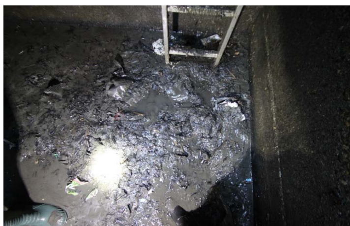
Figure 2 : Trapped pollutants in Sablons basin plenum chamber
