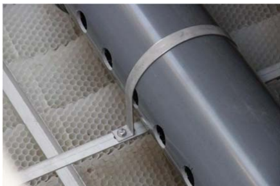
Figure 7 : View of the lamellar blocks lower part
