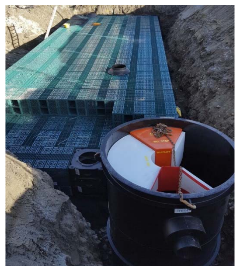
Figure 2 : First Defense® upstream of a Rigofill® system
