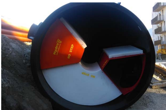
Figure 1 : First Defense®, Ø 1'800 mm treatment flow 90 l/s
