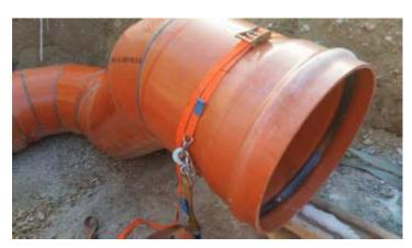
7. Pass a 3<sup>rd</sup> and 4<sup>th</sup> SpanSet<sup>®</sup> in the first 2, on each side of the pipe and along the axes.
