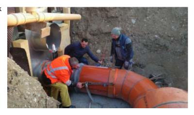
9. Now tighten the 3<sup>rd</sup> and 4<sup>th</sup> SpanSet<sup>©</sup> simultaneously so as to fit the pipe to the mark made in step 2. The fitting is now complete.
