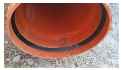
2. Mark the length of the M/F fitting on the smooth end of the pipe to be inserted.
