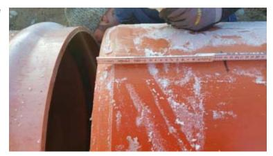
3. Apply soap or petroleum jelly only on the lip of the seal and on the end of the pipe to be inserted (Never use grease, it deteriorates the seal)
