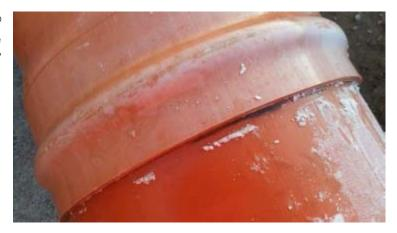
10. Check with a torch that the sealing joint has not come out of its groove and that the pipe is fully fitted.
