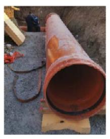
5. Insert the pipe 2-3 cm into the female fitting, stopping just before the seal.
