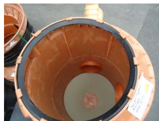
Insertion of the sealing joint on the telescopic reduction cone
