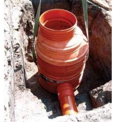
Figure 5 : Laying a room to fill
