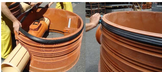
Insertion of the sealing joint (point 4)
